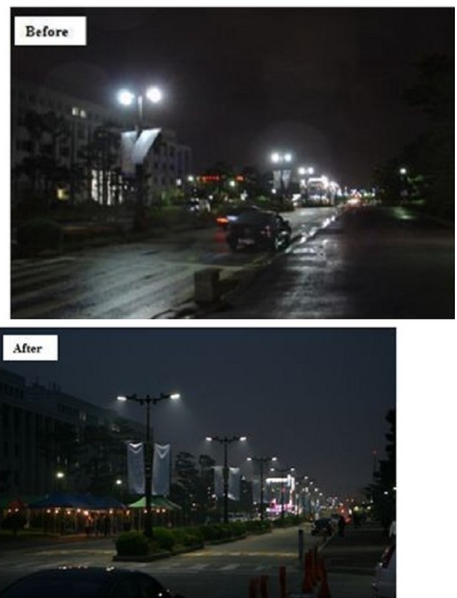
Figure 3.3. Realization of Smart LED lighting system.
