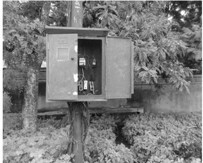
**Figure 1. Normally open distribution point.**
