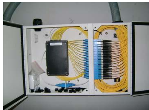
Fig.3 PON Splitter
