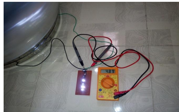
Electricity Generator testing with roof ventilator 7.1
