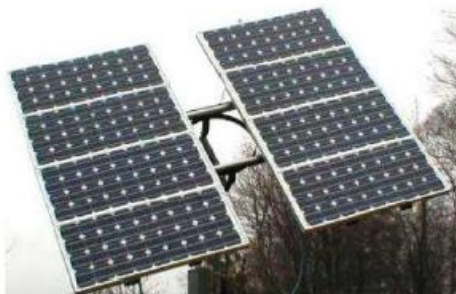
Figure 1.3: dual axis solar tracker
